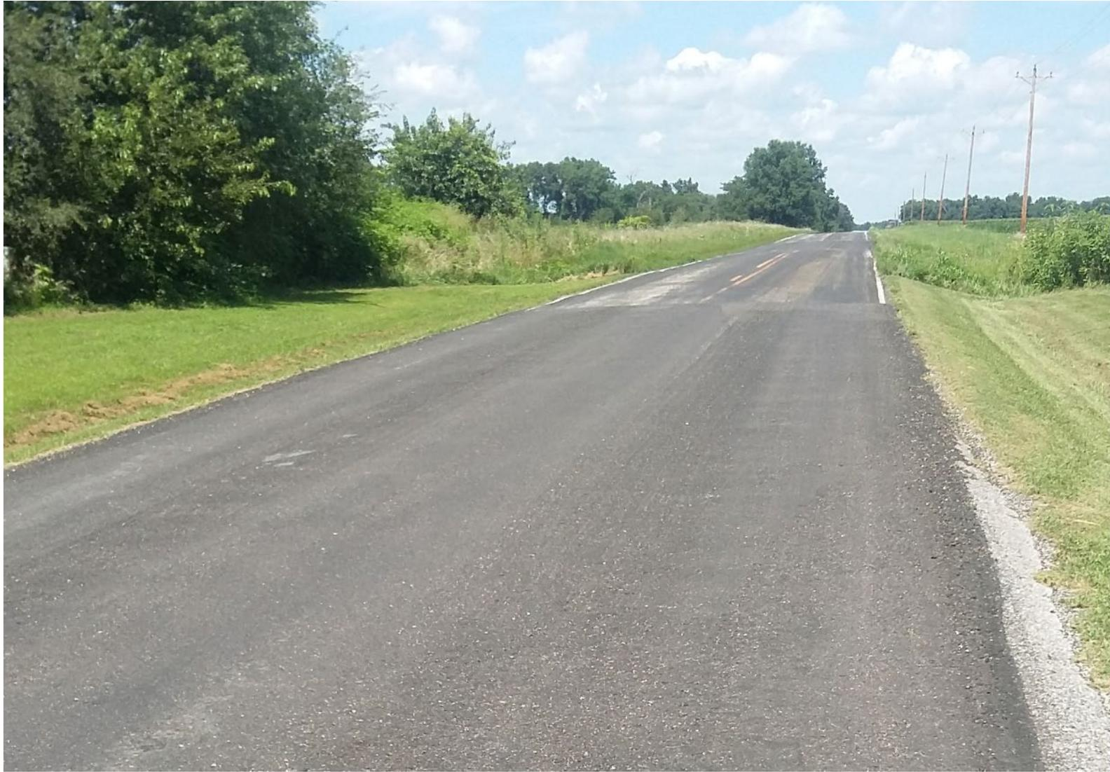
Typical asphalt pavement repair
